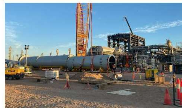
Primary stack positioned for fit up and weld out
